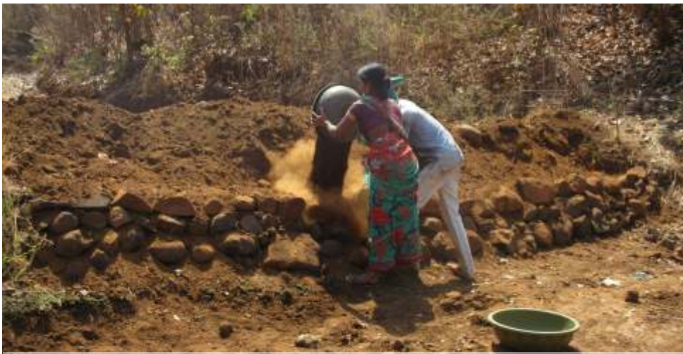
Construction of watershed in Kanur village, Ambernath.
